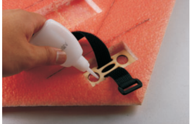
5. Glue the battery velcro by using CA.
