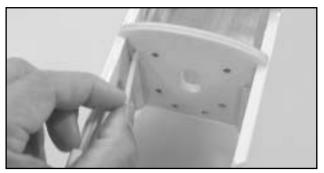
□ Insert the throttle tubing first. It runs along the right side of the fuselage and goes from the up corner of the firewall back through the right hole in the first former and then through the right hole in the second former.
