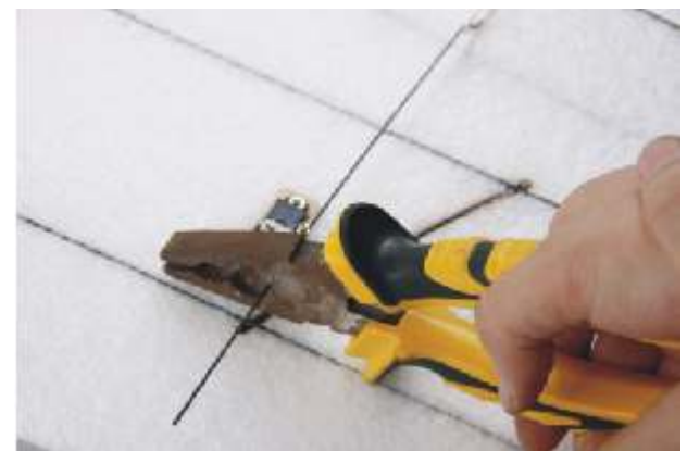
15.Using the pilers to cut off the excess steel wire.
